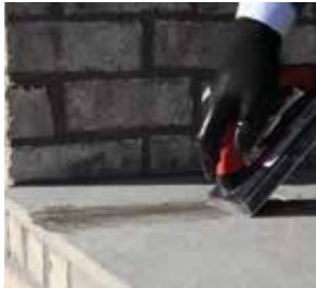
PIC 1. Fill joint with grout.
